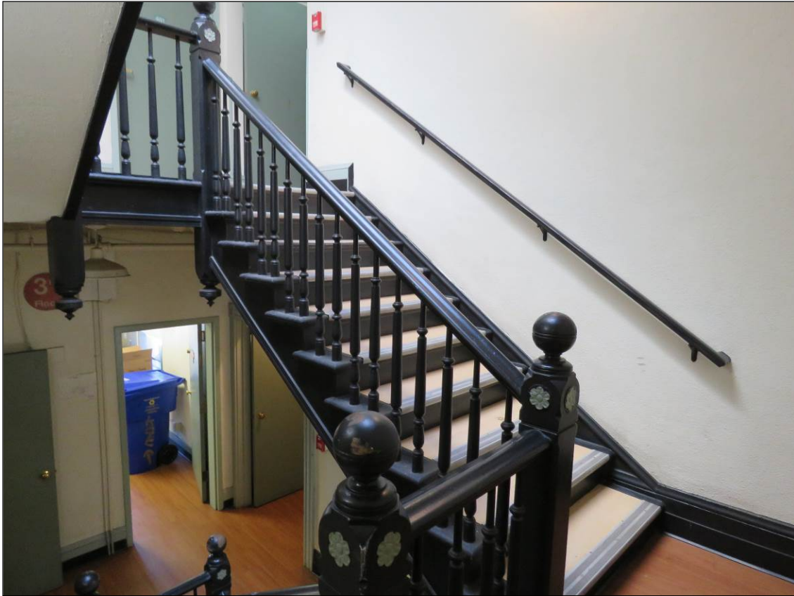
Photograph 7 of 20: OR_MultnomahCounty_GoldenWestHotel_0007 Golden West Hotel primary staircase, camera facing northeast.
