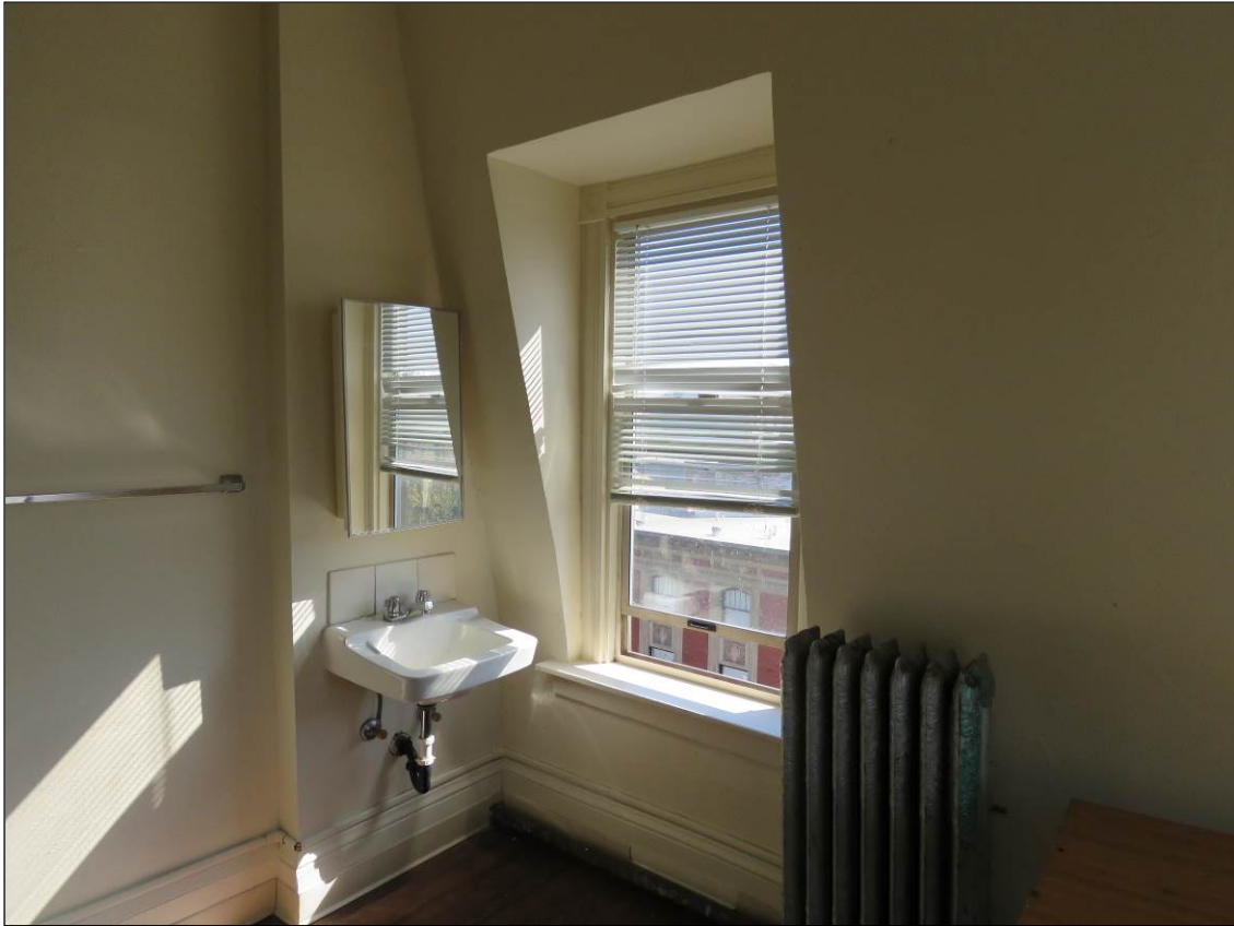
Photograph 15 of 20: OR_MultnomahCounty_GoldenWestHotel_0015 Representative view of residential room in Golden West Hotel, camera facing northeast.
