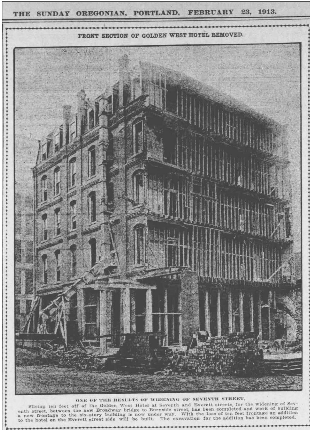
Figure 14: "Front Section of Golden West Hotel Removed," Sunday Oregonian (Portland, OR), February 23, 1913.
