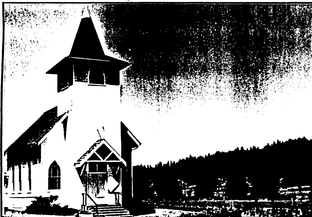
Fig. 436 Gothic Church Territorial Road Corridor
