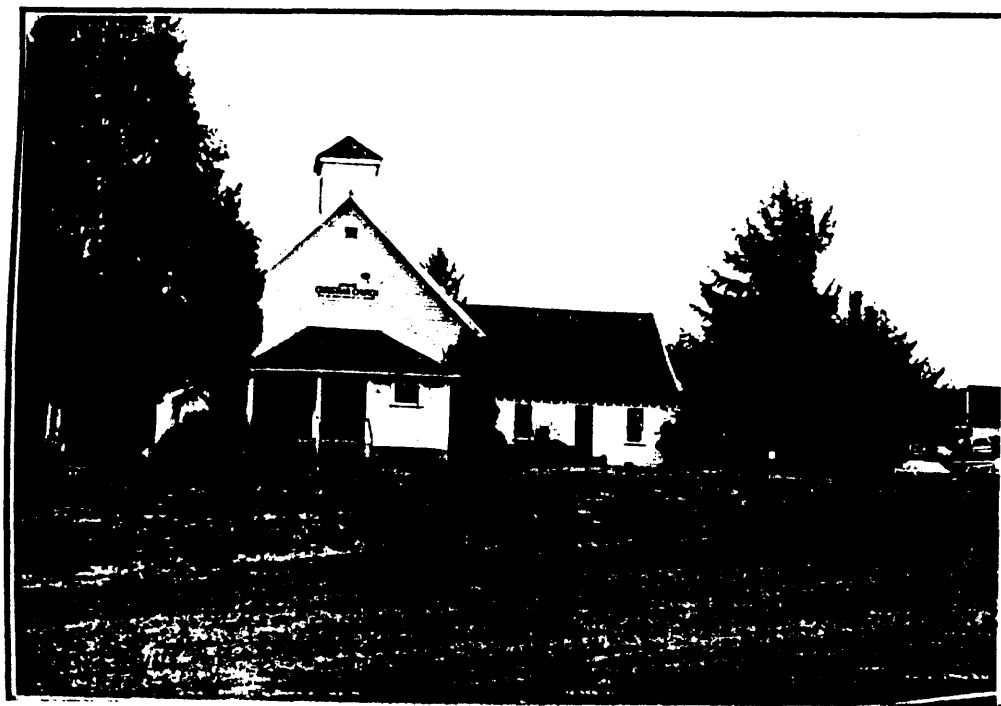
Fig. 456 Gothic Church Territorial Road Corridor
