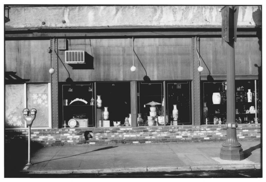
Photograph 5 of 6 View of the 3rd Avenue storefront, showing the structural I-beam columns, with the display window infill; plywood and brick veneer covering original storefront material still existing.
