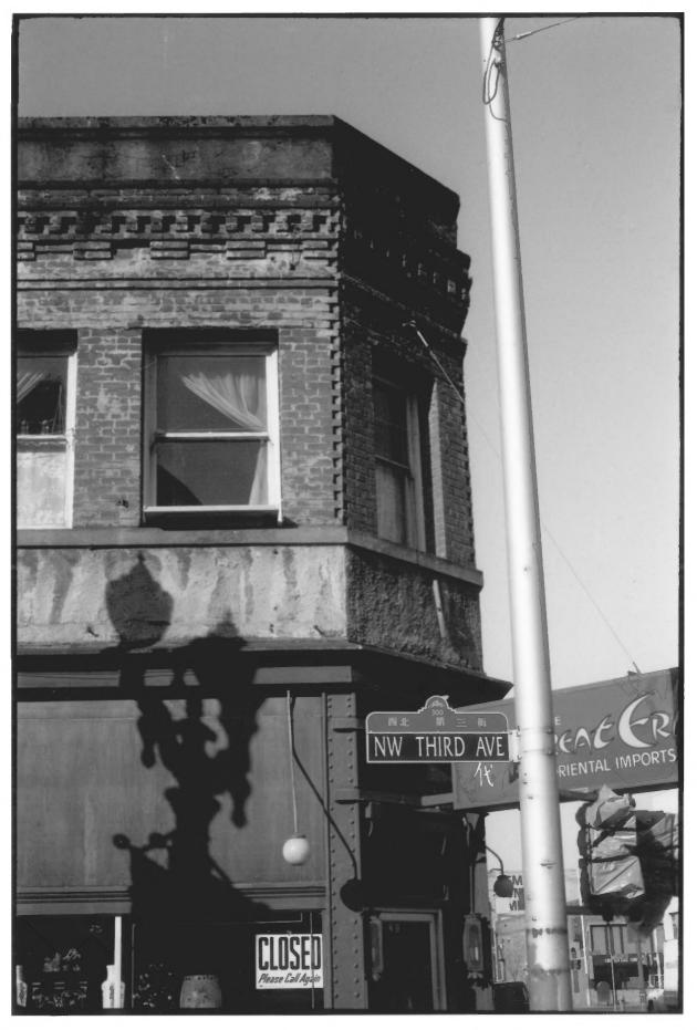
Photograph 2 of 6 Close up of corner entrance and relationship of the steel I-beam ground floor store fronts and the upper floor brick. Looking south.
