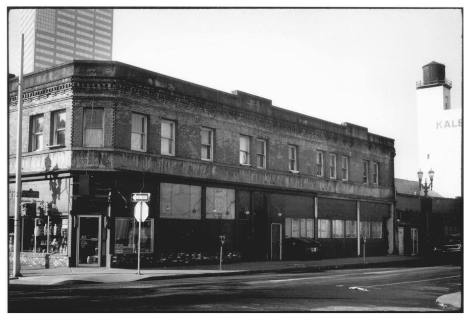
Photograph 6 of 6 The north elevation (Everett Street) looking south, showing the articulated parapet wall, original entrances including the exterior basement entrance location at mid point of the elevation.
