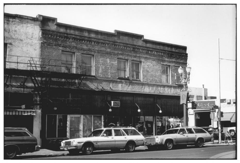
Photograph 4 of 6 The east elevation on 3rd Avenue, looking west, showing the two story air rights development; articulated parapet wall, stone coping and decorative brick work, stringcourse.
