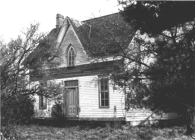
4 of 11 NOV 6 1980 North (front) and west elevations. Scar on facade is from second porch added in early 20th century. Gothic door was shortened for use as window as a result of this change.
