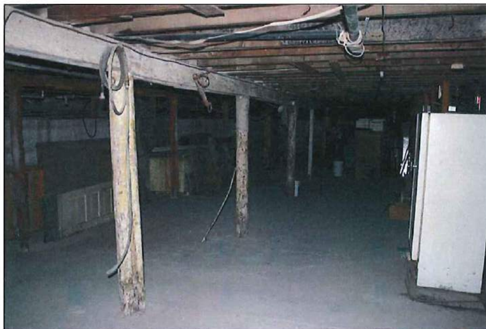
Photo 16 of 16: Showing the basement, July 2013
