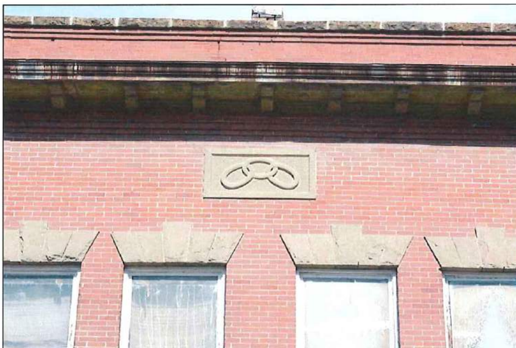
Photo 2 of 16: West (front) elevation detail showing the Odd Fellows symbol, cornice, and lintel looking east, July 2013
