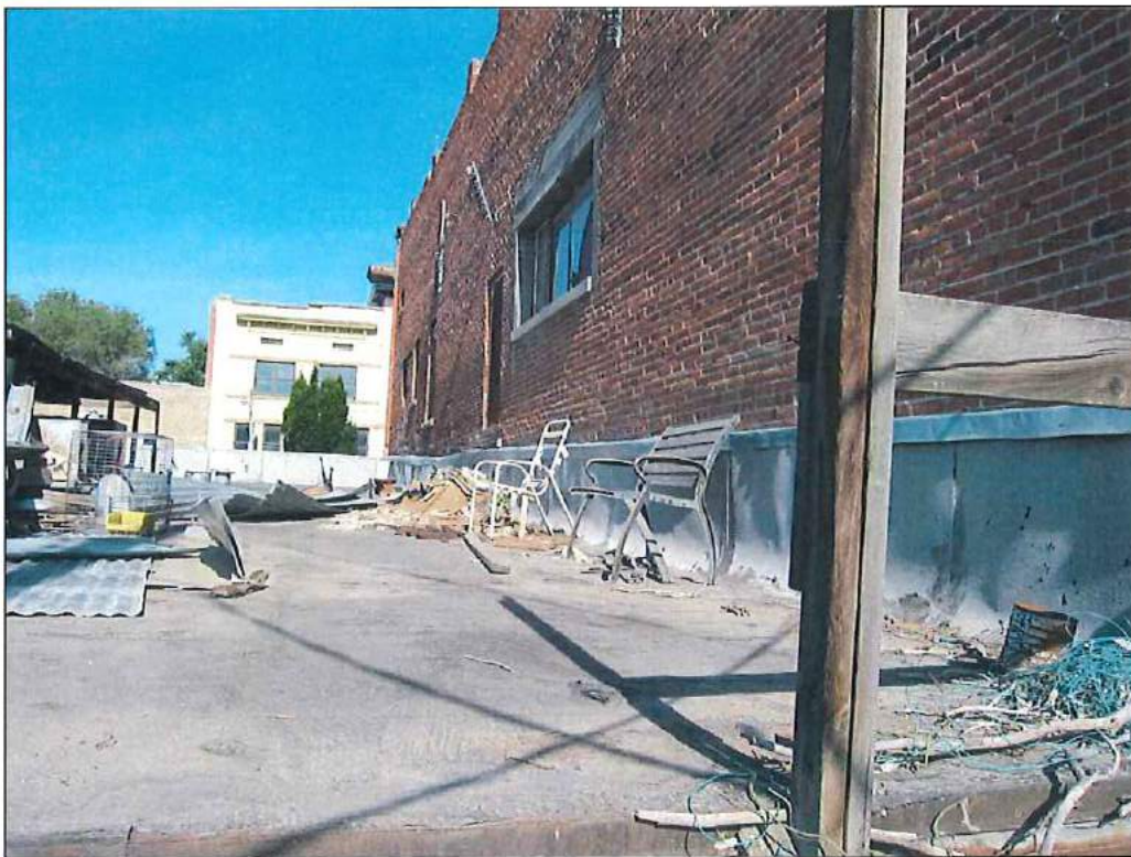
Photo 10 of 16: South elevation showing second story, looking northwest, July 2015
