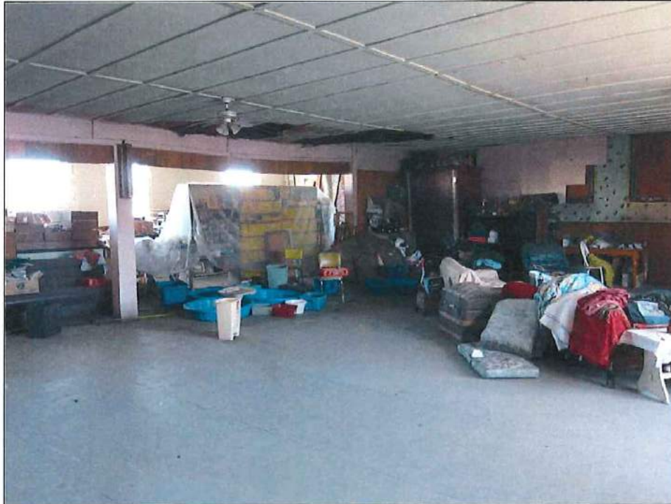
Photo 13 of 16: Showing IOOF meeting hall with space separated by columns, looking northeast, August 2010
