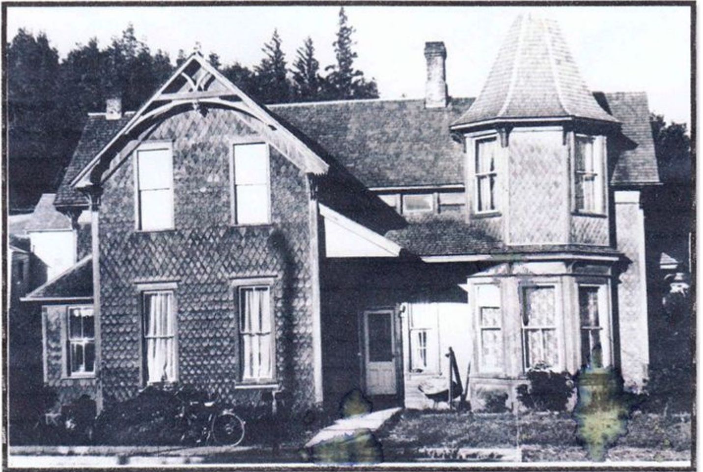
Figure 11: Peter John Lindberg House (c.1960), looking west.
