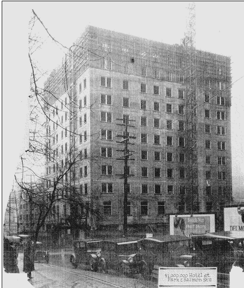
Figure 8: Looking NE from SW, Heathman Hotel, under construction, circa 1925
