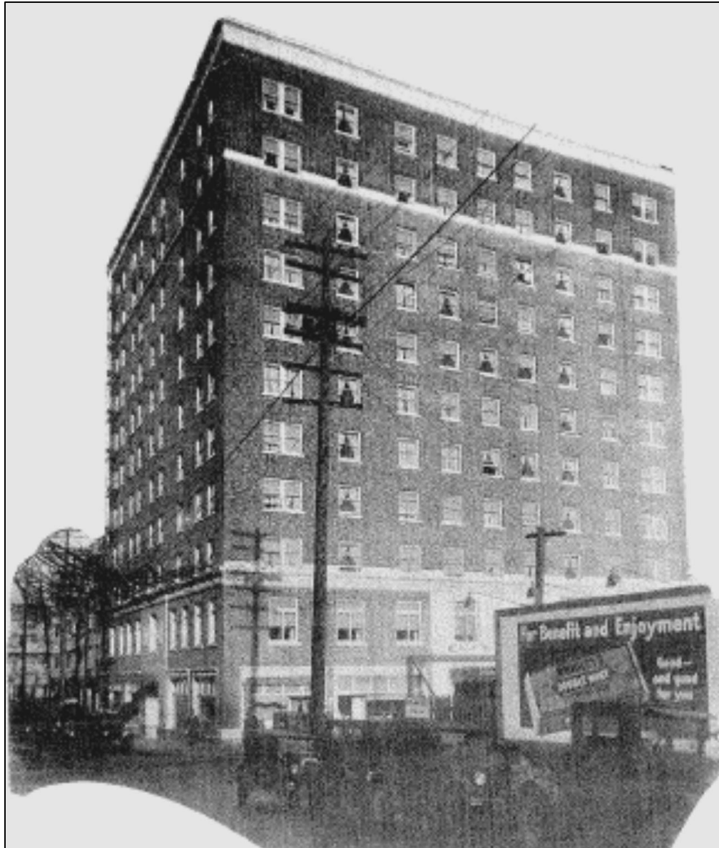
Figure 9: Looking NE from SW, Heathman Hotel, after construction, 1926
