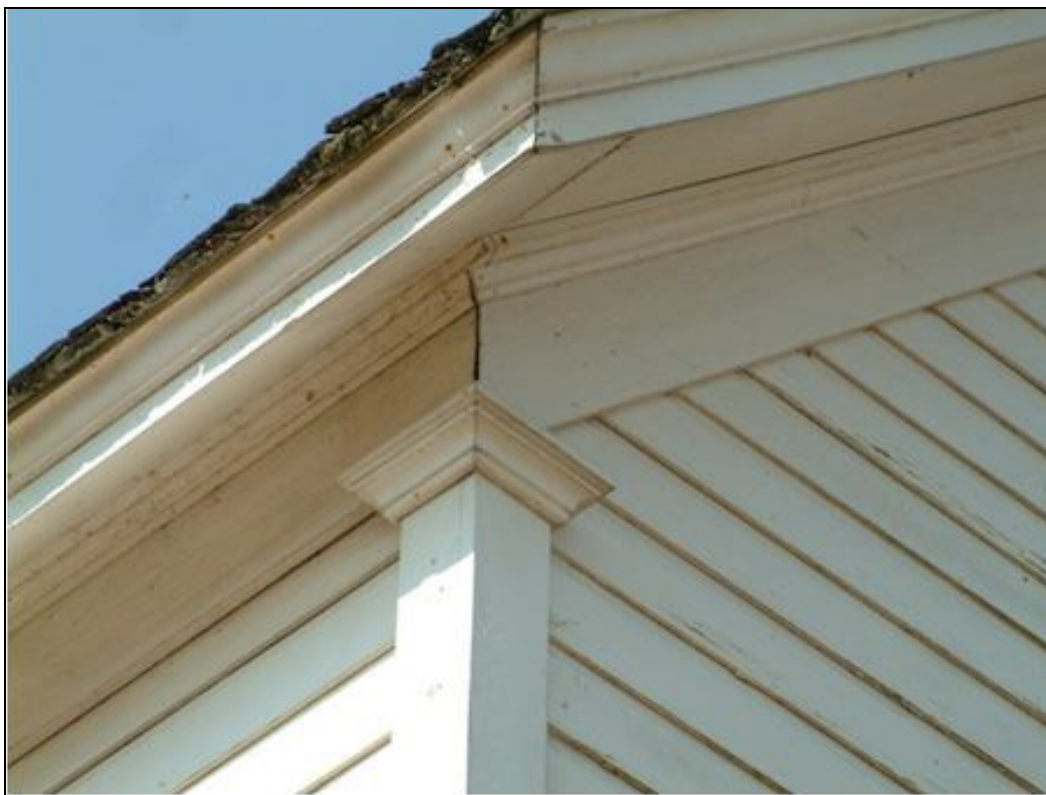
Photo 9 of 12: Detail of cornerboard and cap, frieze and eave.
