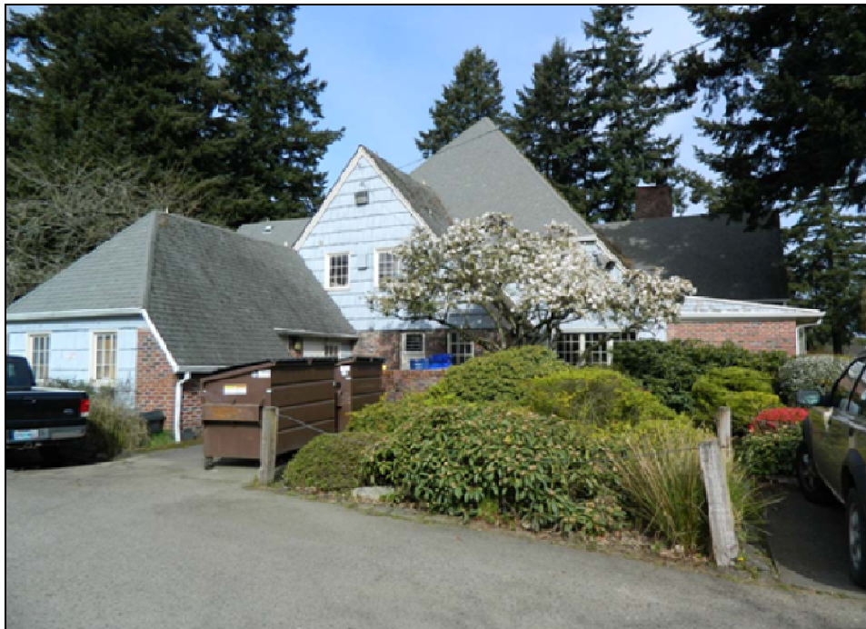
Photo 4 of 12: (OR_MultnomahCounty_RoseCityGolfClubhouse_0004) Southeast façade, looking northwest.
