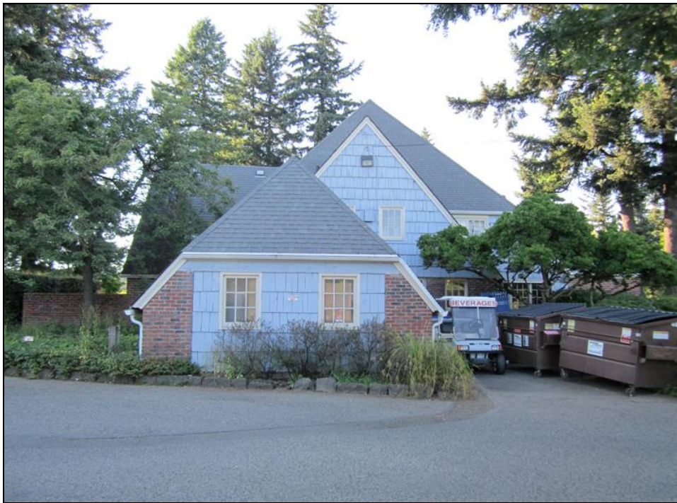
Photo 6 of 12: (OR_MultnomahCounty_RoseCityGolfClubhouse_0004) Southeast façade, looking northwest.
