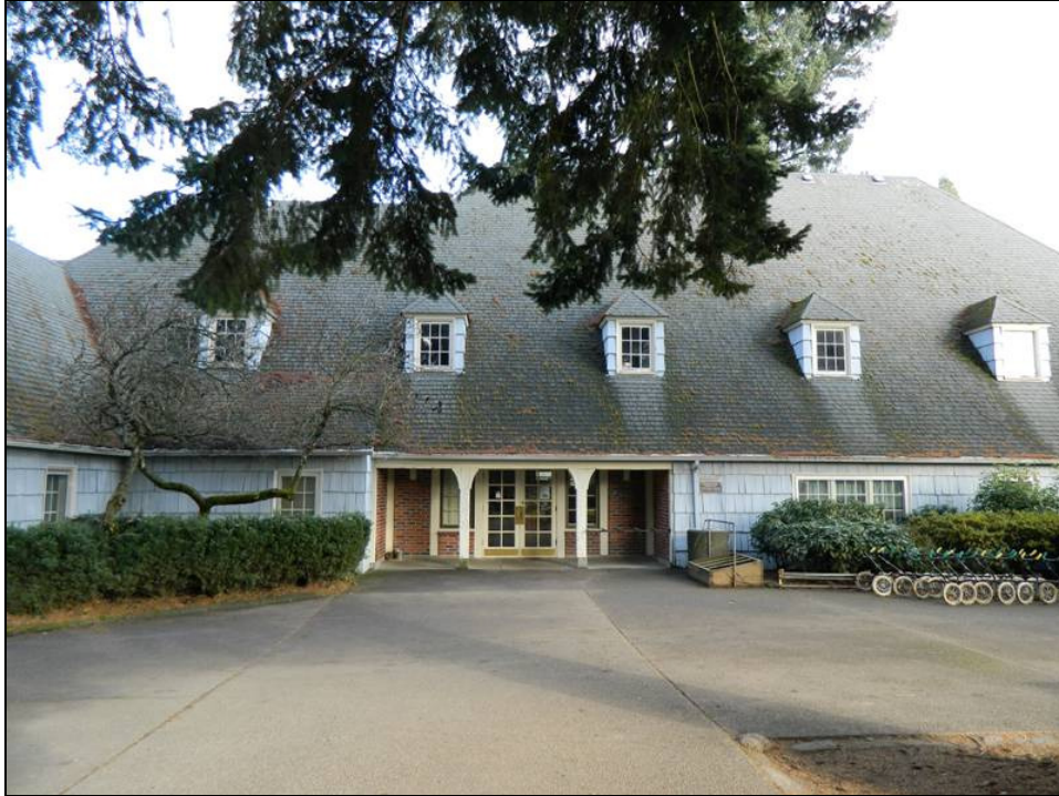
Photo 5 of 12: (OR_MultnomahCounty_RoseCityGolfClubhouse_0003) Southwest façade, looking northeast.
