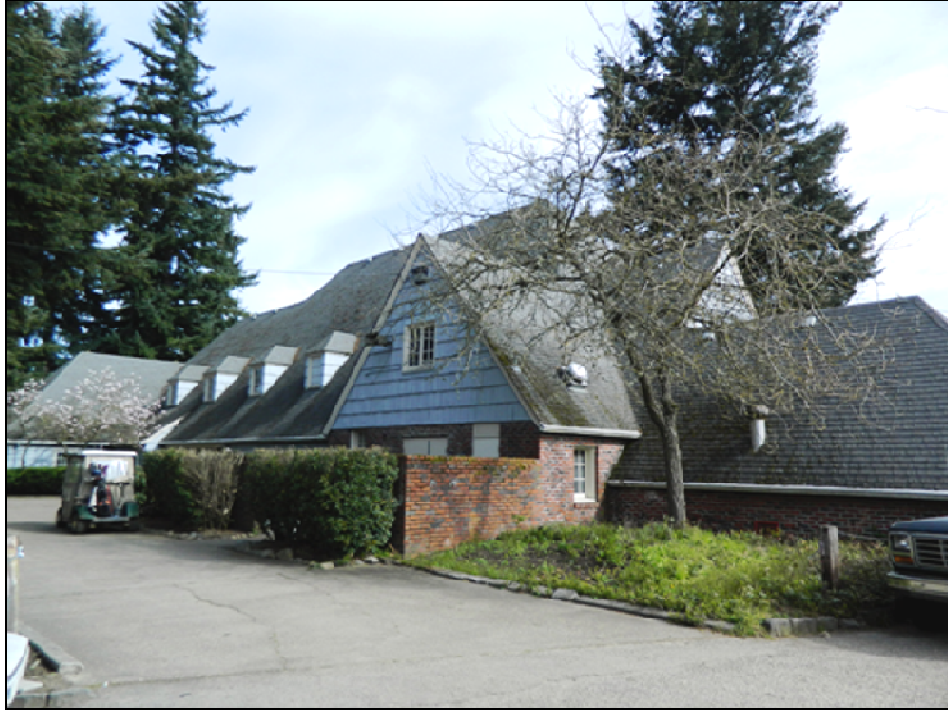
Photo 3 of 12: (OR_MultnomahCounty_RoseCityGolfClubhouse_0003) Southwest façade, looking northeast.
