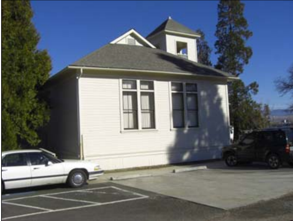
Photo 3 of 13: OR_JacksonCounty_TalentElementarySchool_0003 West-facing [Side] elevation, looking SE, from parking area
