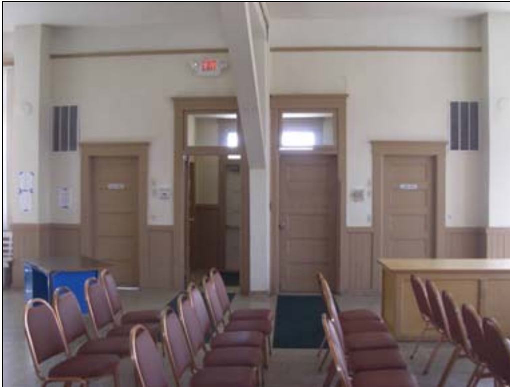
Photo 9 of 13: OR_JacksonCounty_TalentElementarySchool_0009 INTERIOR: Entry doors, restroom doors, looking South from main meeting space
