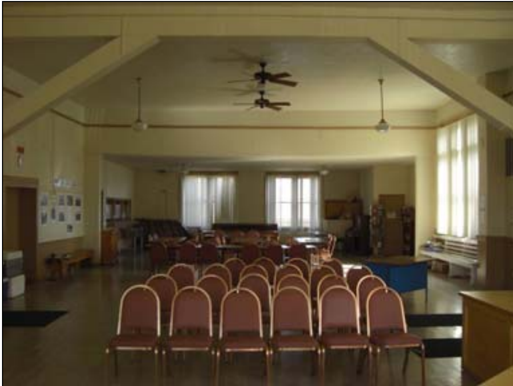
Photo 11 of 13: OR_JacksonCounty_TalentElementarySchool_0011 INTERIOR: Main meeting space, looking East, toward addition
