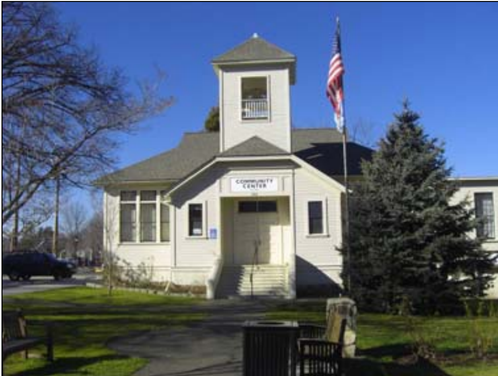
Photo 1 of 13: OR_JacksonCounty_TalentElementarySchool_0001 South Facing [Front] elevation, looking N, from Main Street.
