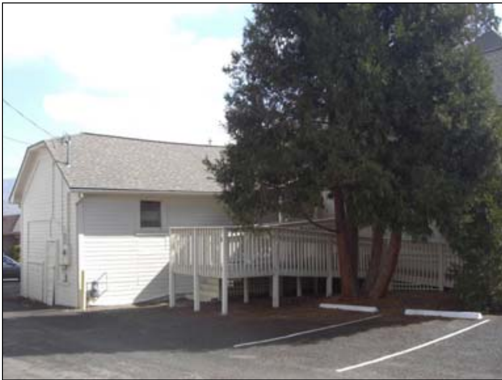
Photo 4 of 13: OR_JacksonCounty_TalentElementarySchool_0004 Rear, "dining room" storage area/ADA-ramp, looking SE, from parking area
