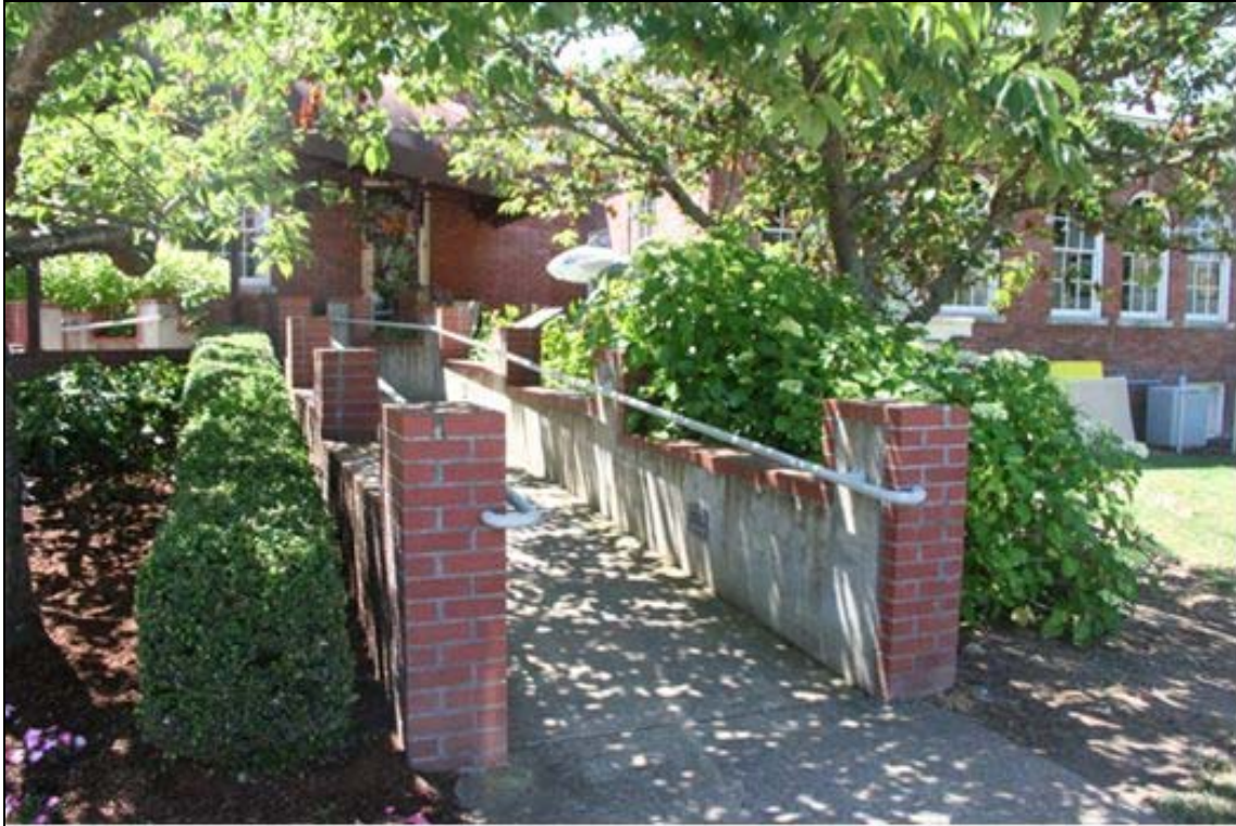
Photo 5 of 16: OR_DouglasCounty_ORStateSoldiersHomeHospital _0005 North façade entrance access ramp, looking southwest
