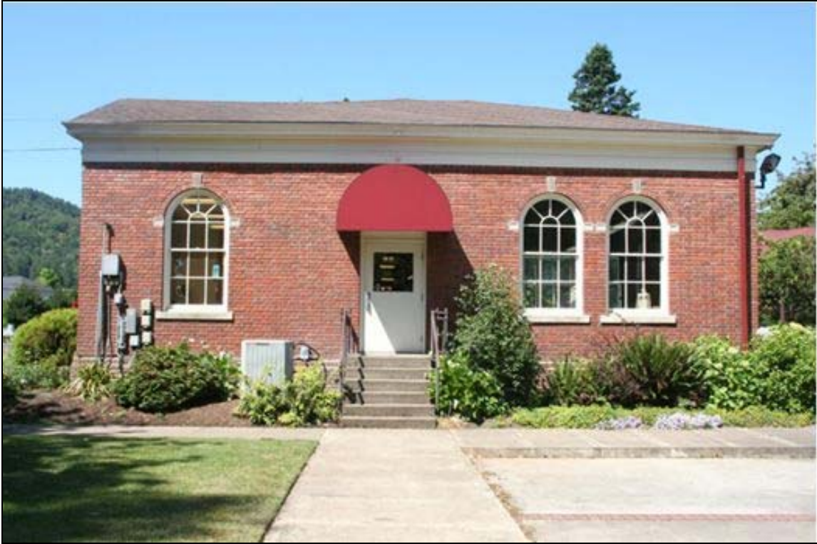
Photo 3 of 16: OR_DouglasCounty_ORStateSoldiersHomeHospital _0003 East façade, looking west
