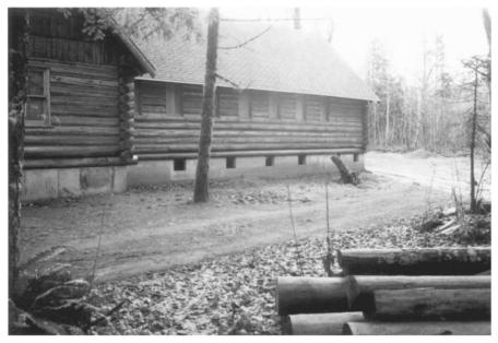
NORTH SIDE GRADUAL TAPER OF BACKFILL WILL FXTENS PAST NORTH SIDE OF DRIVE TO Avoid Monthee LOOK AND PROUTDE BRITER DRAINAGE FOR TBULLDING AND DRIVE. St. John the prompetit Roman Carhalie Church
