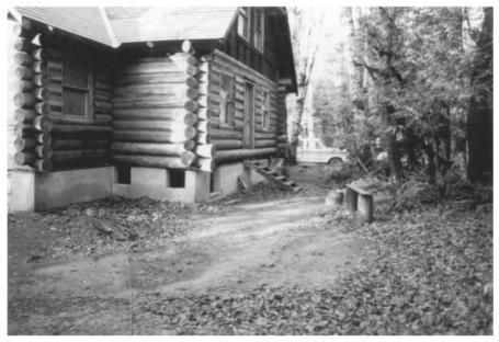
FAST FND NOTE THAT EXISTING EAST GRADE LENDS ITSELF MILELY TO ABOUT 19" OF BACKFILL TO MAKE AREA LEVEL, THIS END AND SOUTH SIDE WERE EXCAUATED TO CLEAR A LEVEL AREA FOR BUILDING. pt. Jul The Everyelist Roman Catholic Church Clockamar a, Olegon
