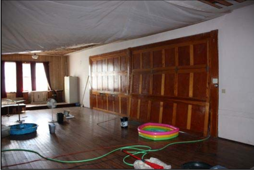
Photo 9 of 16: OR_WallowaCounty_EnterpriseIOOFHall_DowntownEnterpriseMPD_0009 Looking southeast at the lodge hall's hinged partition panel doors.
