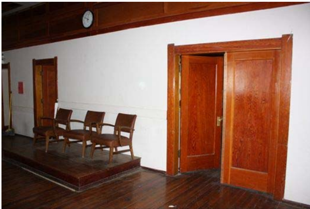
Photo 10 of 16: OR_WallowaCounty_EnterpriseIOOFHall_DowntownEnterpriseMPD_0010 Doors to the paraphernalia room in the west wall of the lodge hall. Panels above open into the balcony.
