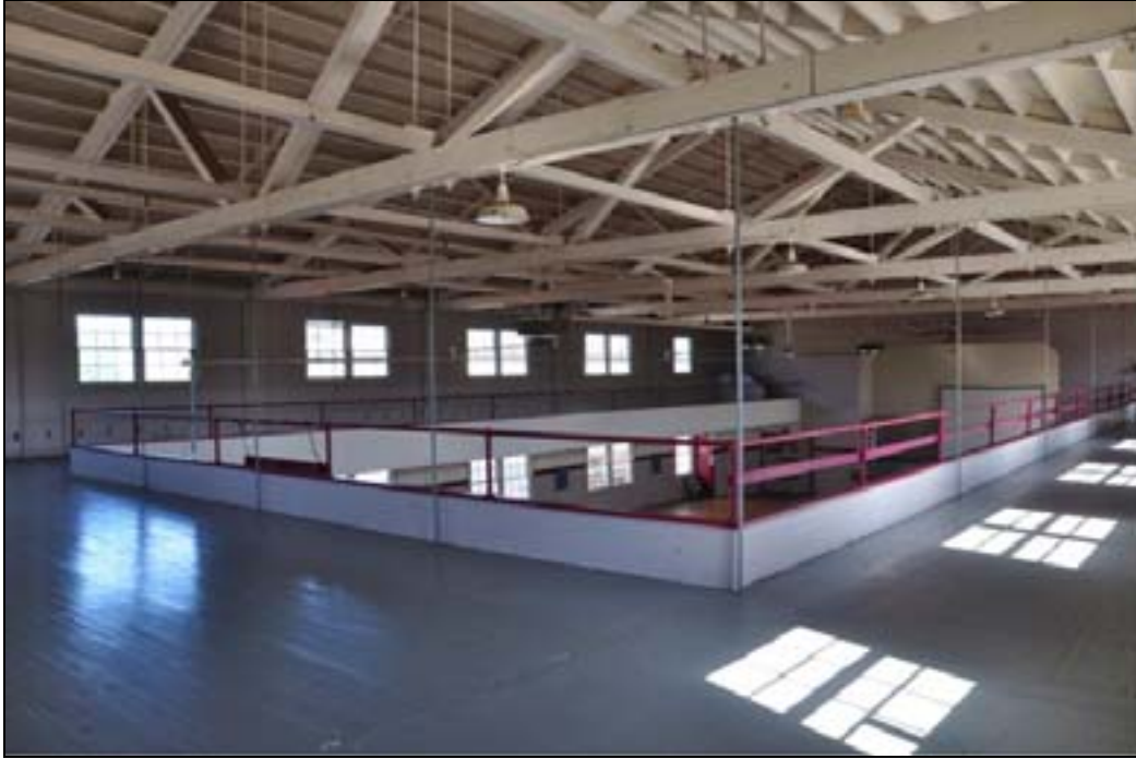
Photo 11 of 22: OR_LaneCounty_CottageGroveArmory_0011.tif Top floor, balcony from lobby. Looking northwest.
