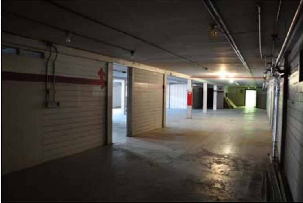
Photo 21 of 22: OR_LaneCounty_CottageGroveArmory_0021.tif Basement, multi-purpose room. Looking north.
