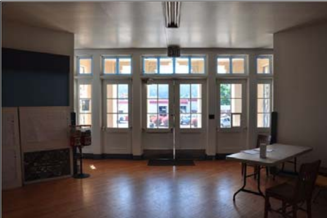
Photo 14 of 22 OR_LaneCounty_CottageGroveArmory_0014.tif Main floor, lobby. Looking southeast.
