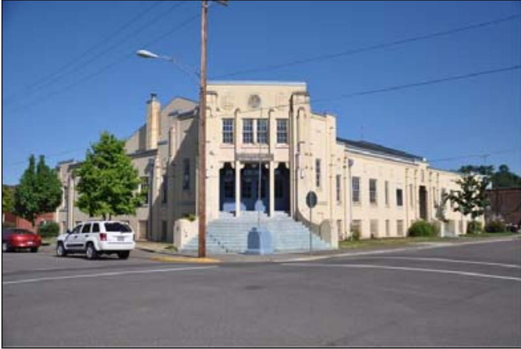
Photo 1 of 22: OR_LaneCounty_CottageGroveArmory_0001.tif Southeast entrance tower and east and south facades. Looking northwest.
