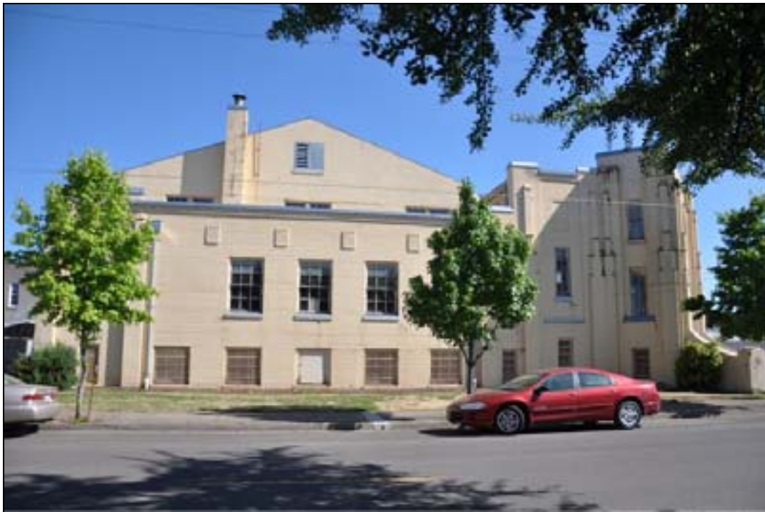
Photo 8 of 22: OR_LaneCounty_CottageGroveArmory_0008.tif South façade. Looking north.
