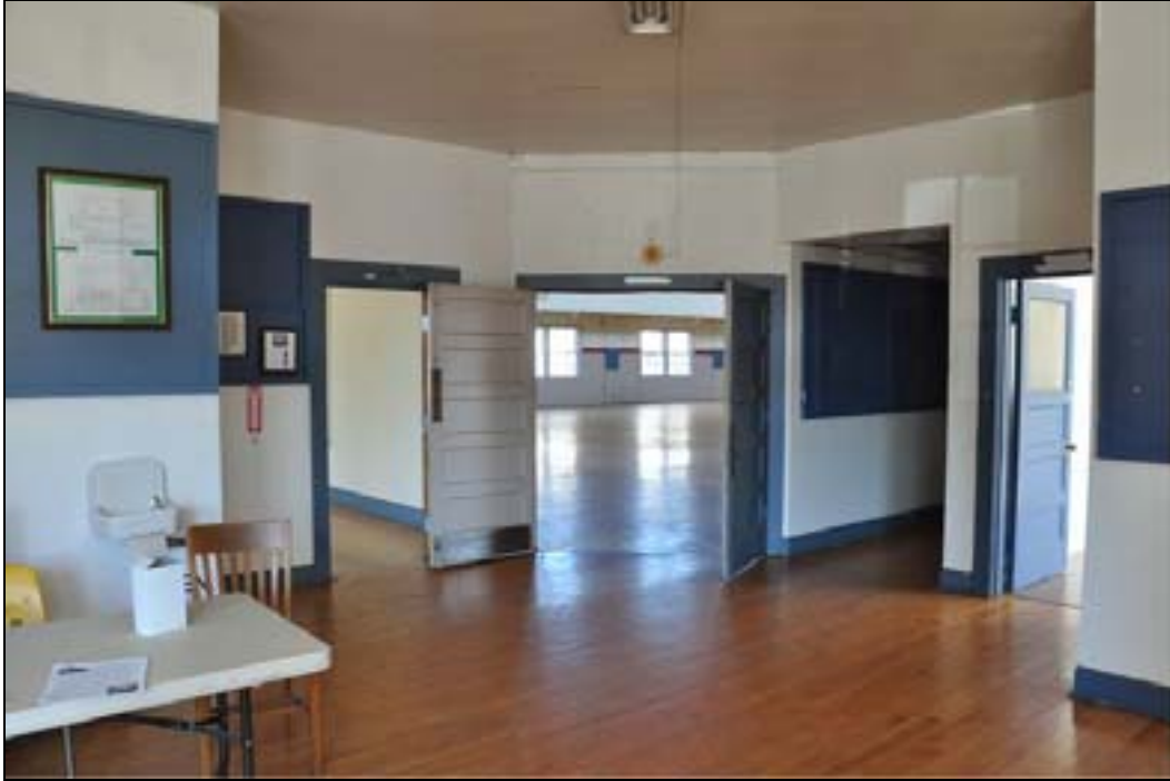
Photo 15 of 22: OR_LaneCounty_CottageGroveArmory_0015.tif Main floor, lobby. Looking northwest.
