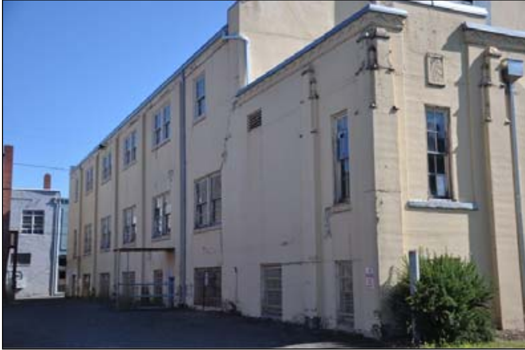
Photo 9 of 22: OR_LaneCounty_CottageGroveArmory_0009.tif West façade. Looking northeast.
