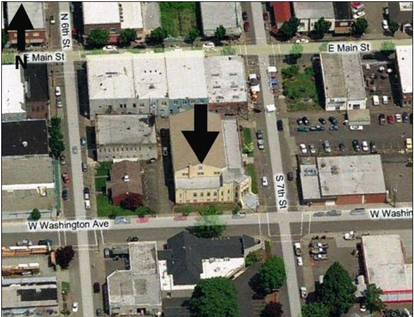
Figure 2: Aerial view of Cottage Grove Armory and surrounding block, 2011. Location of Cottage Grove Armory marked with arrow.
