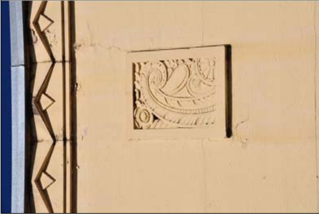
Photo 7 of 22: OR_LaneCounty_CottageGroveArmory_0007.tif Detail of Terracotta tile and chevron frieze on east façade. Looking west.
