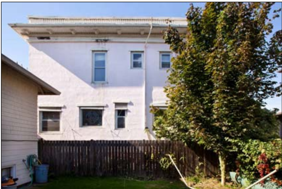
4 of 14: OR_MultnomahCounty_GeorgeWandHettyABowersHouse_0004 East façade, camera facing west.
