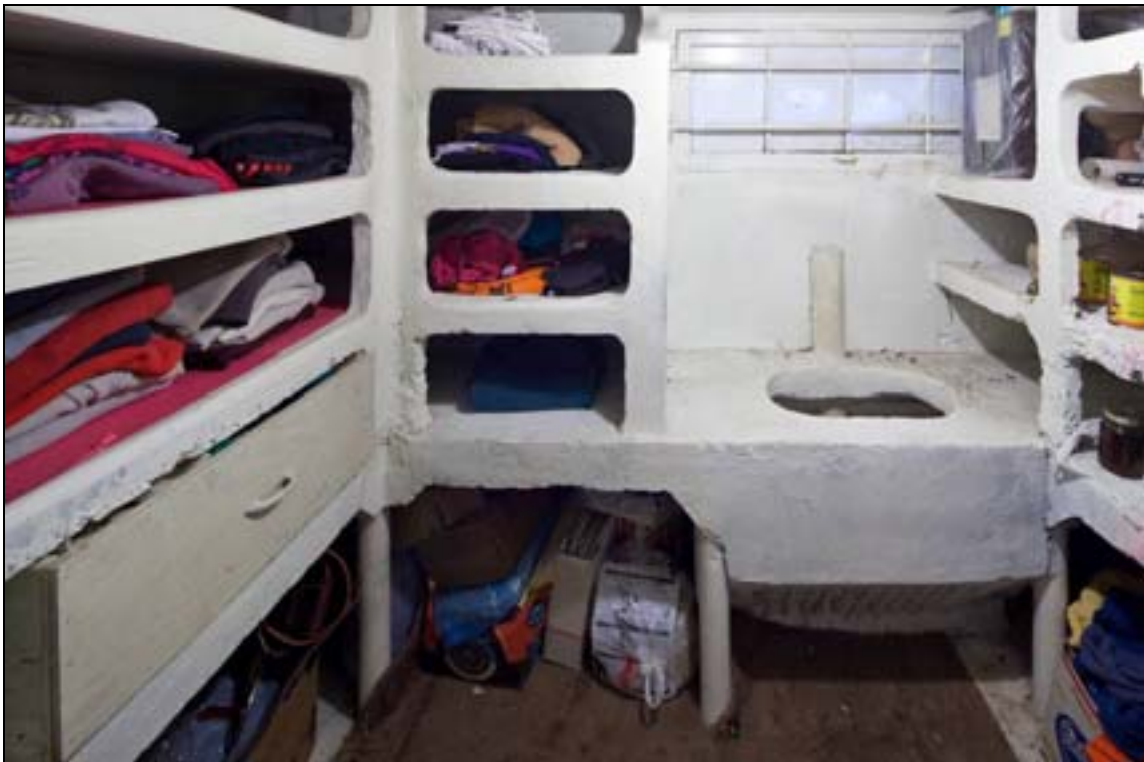
12 of 14: OR_MultnomahCounty_GeorgeWandHettyABowersHouse_0012 Basement Fruit room, camera facing east.
