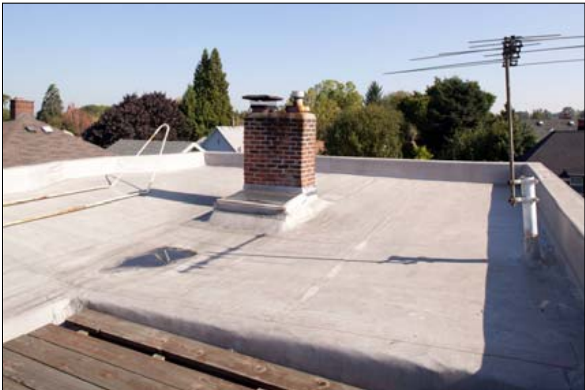
6 of 14: OR_MultnomahCounty_GeorgeWandHettyABowersHouse_0006 Rooftop, camera on roof facing northeast.
