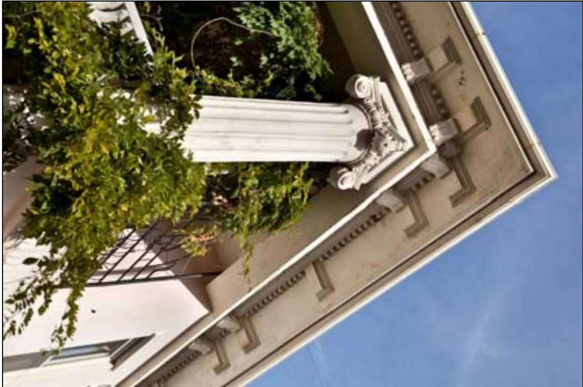
3 of 14: OR_MultnomahCounty_GeorgeWandHettyABowersHouse_0003 Detail of column, capital, and entablature at second floor porch. Camera facing northeast, taken from below on the sidewalk.
