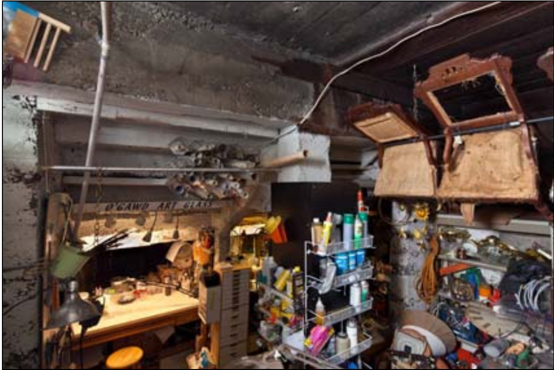
13 of 14: OR_MultnomahCounty_GeorgeWandHettyABowersHouse_0013 Basement below entry porch and stairs, camera facing northwest.
