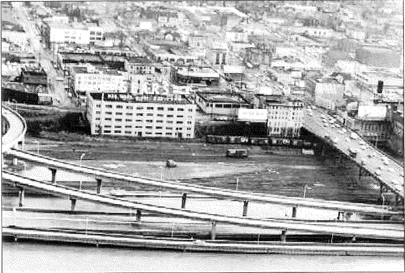
Figure 16: Ira F. Powers Furniture Company Warehouse and Factory (Sears) Aerial looking east from west c. 1950, Oregon Historical Society
