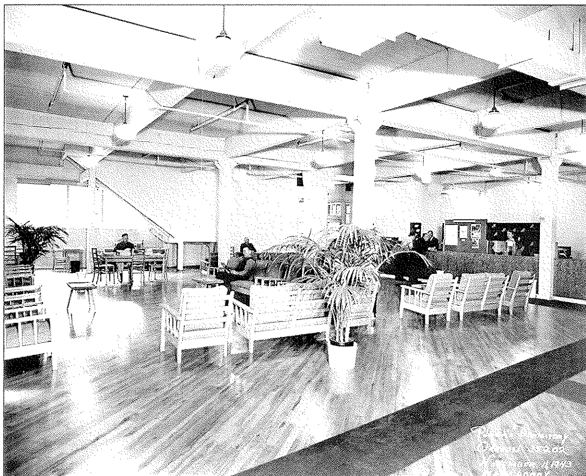
Figure 13: Powers Dormitory Main Lobby, Looking SE, November 11, 1943 (Portland City Archives, A2001-0.25.379)
