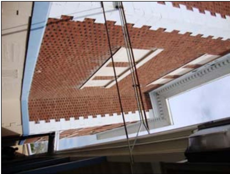
Photo 6 of 13: (OR_UmatillaCounty_CentralSchool_0006) Exterior View: South elevation, looking northeast
