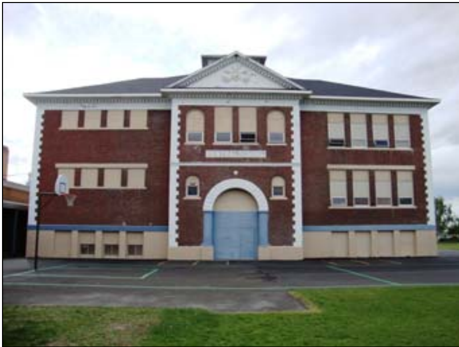
Photo 1 of 13: (OR_UmatillaCounty_CentralSchool_0001) Exterior View: Main Façade, east side, looking west
