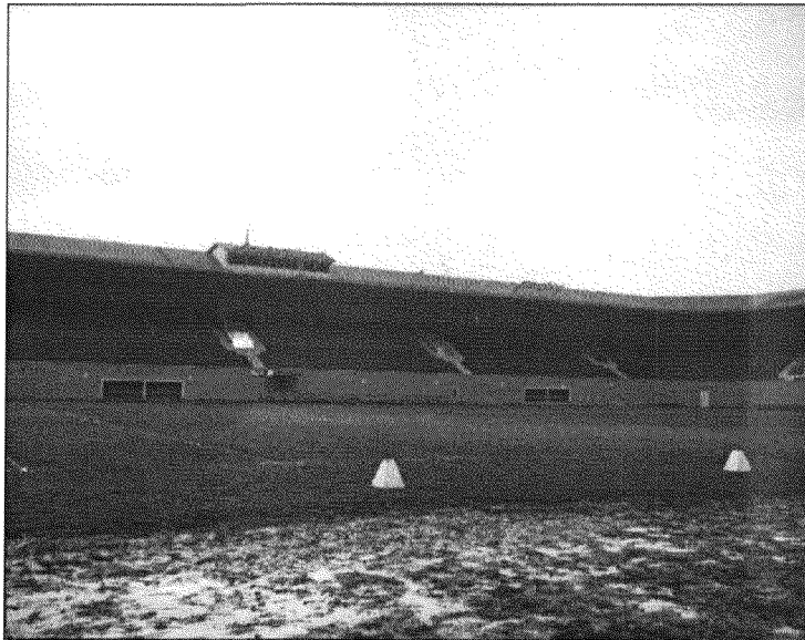
Figure 13: Eugene Civic Stadium, circa 1950. Note the lines on the field (for football) and the central entrance on the 50-yard line. This photo also shows a press box on the roof of the Grandstand, which is believed to have been removed during the 1969 conversion of the stadium to a baseball facility for the Eugene Emeralds. Courtesy of the Lane County Historical Museum.
