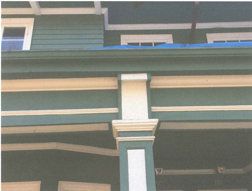
Front Porch/Balcony Detail
