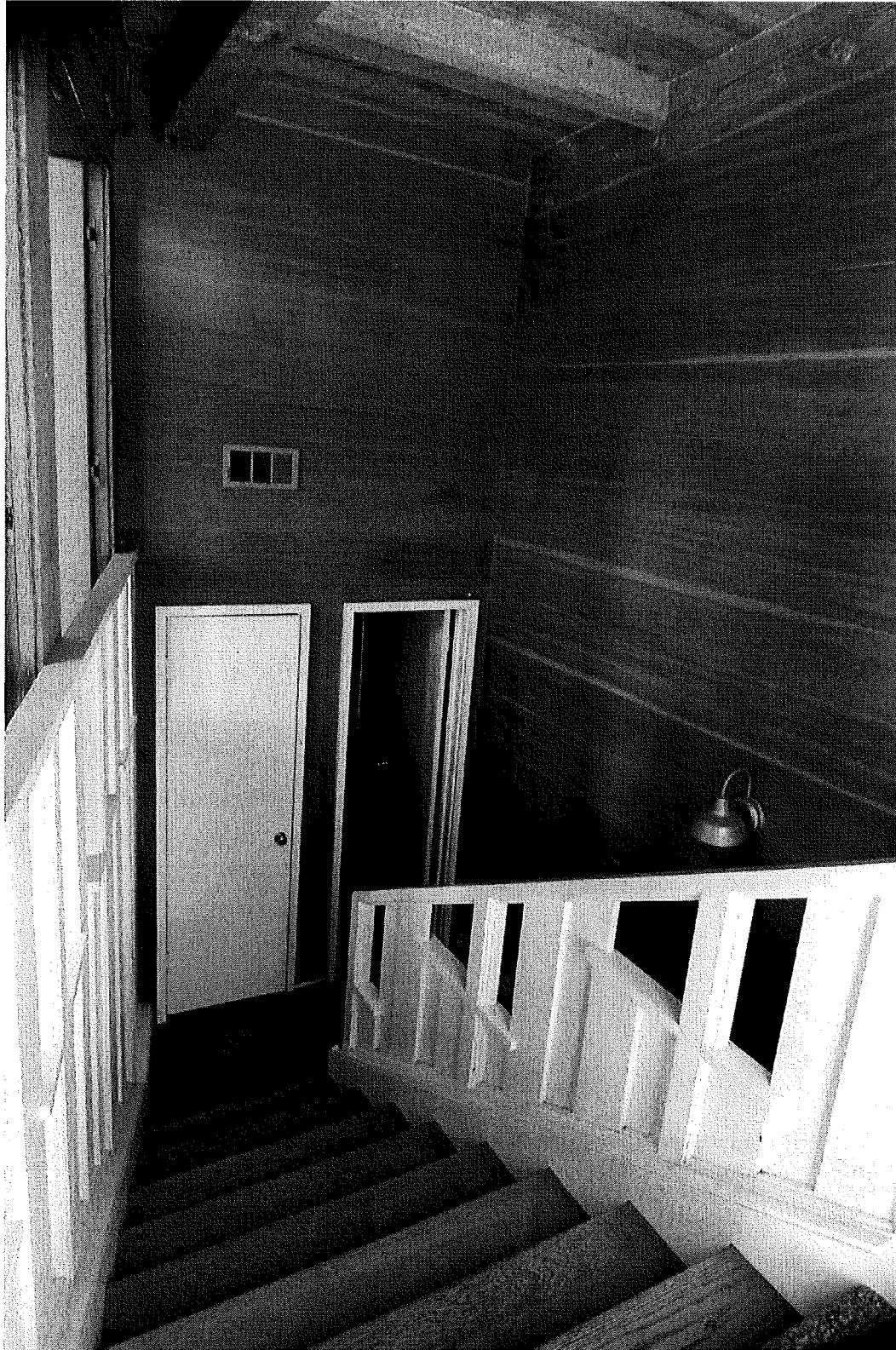
Photograph 6: Sallie Wagner & William J. Lippincott House, Interior, Stairwell (March 2014)
