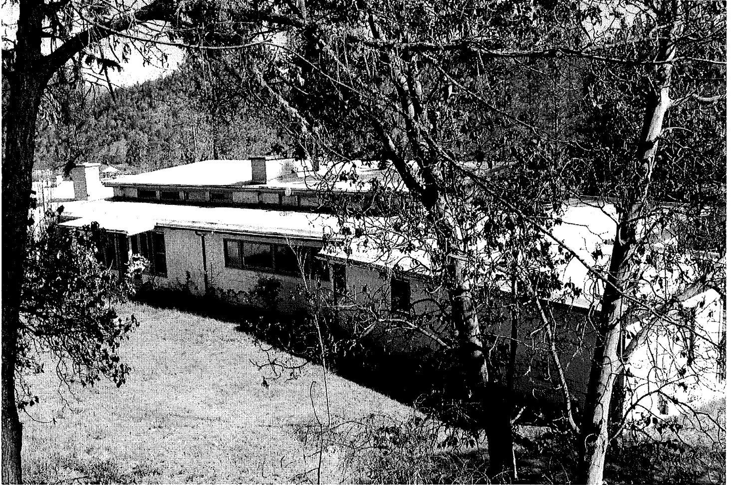
(note scorched tree from June 2013 fire at extreme left)
