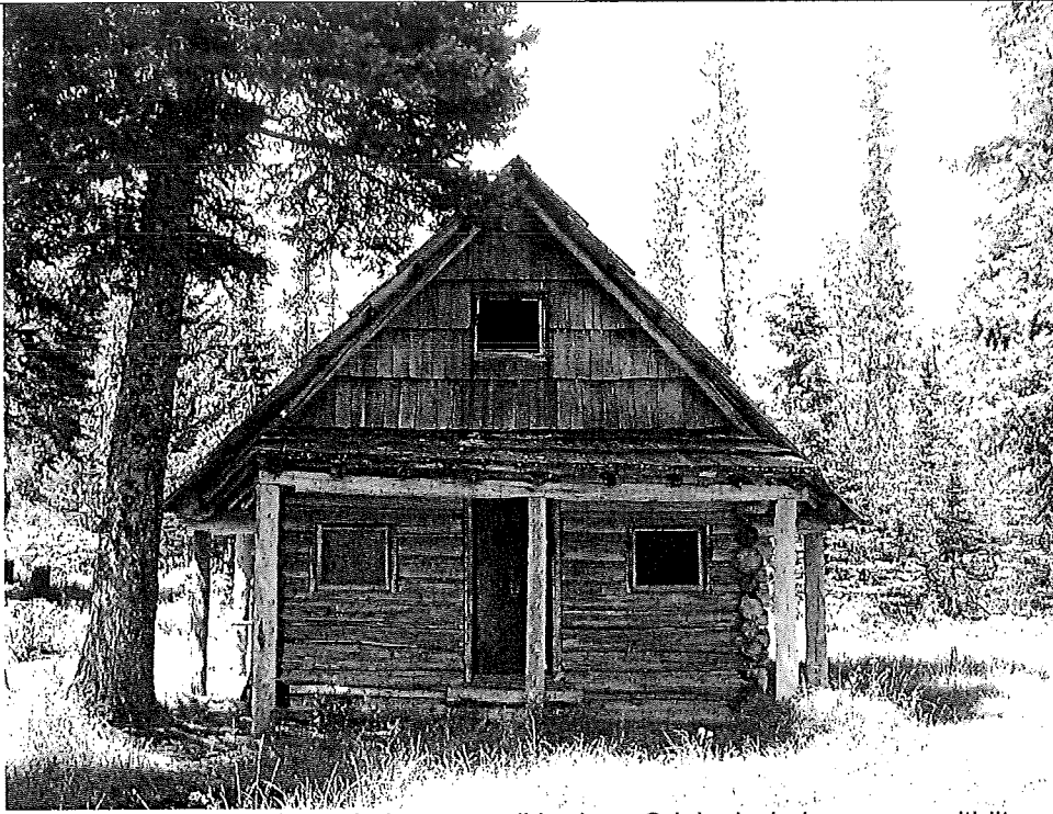
Figure 2. East elevation, windows are all broken. Original windows are multi-lites, three-over-three. Photo taken August 2013.
