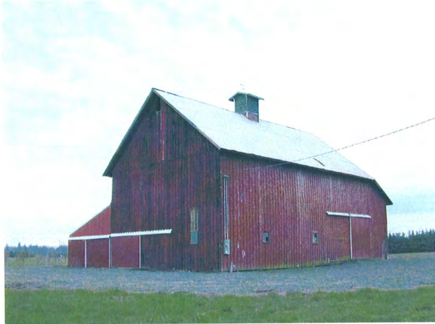
View: Stipp barn, east and north (front) elevations.
