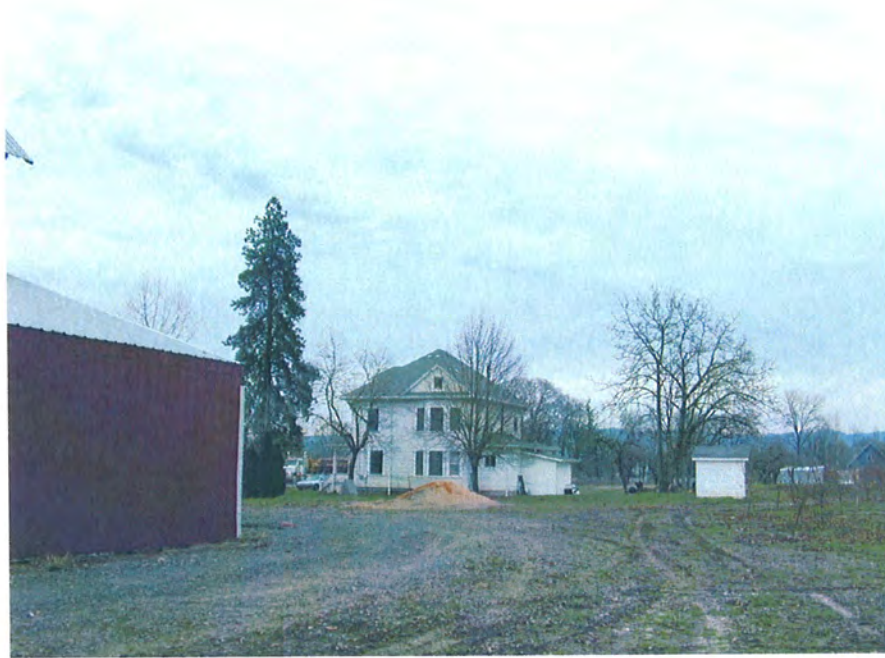
View: West elevation of the Stipp house, also showing the barn on the left and the small, modern pump house to the right. View to east.
