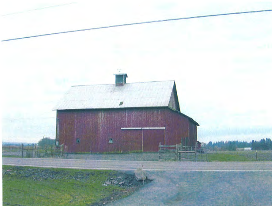
View: Stipp barn, north (front) elevation from across S. Molalla Avenue.
