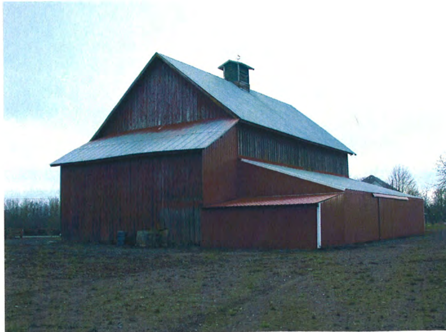
View: Stipp barn, west and south (rear) elevations
