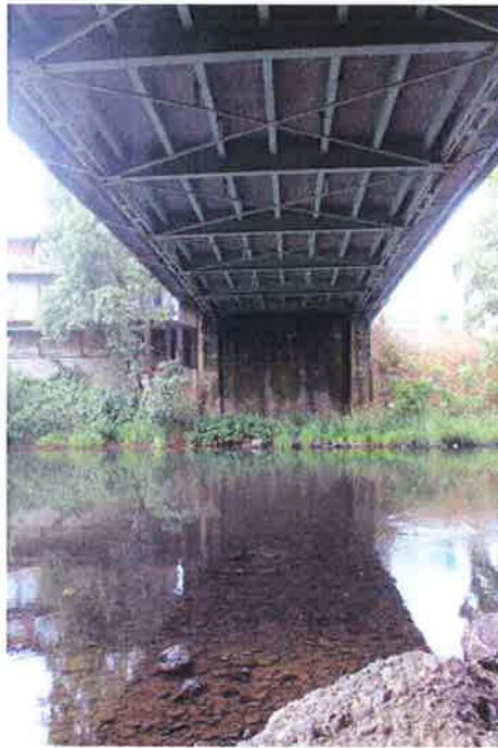
Figure 11.: Sheridan Bridge, Substructure, Looking North, across S. Yamhill River, July 2011
