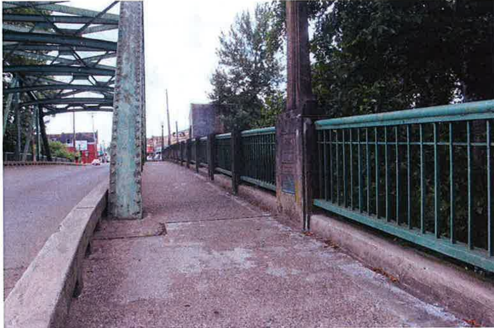
Figure 9.: Sheridan Bridge, Looking South, showing outer bridge rail and plaques, July 2011
