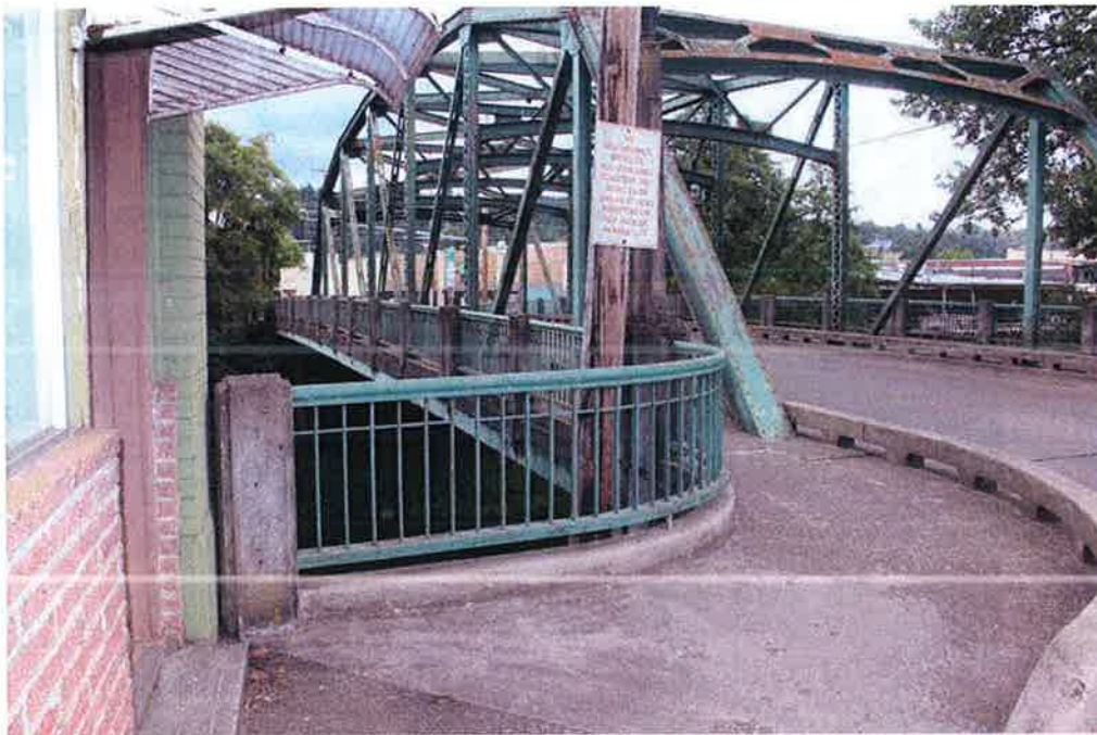
Figure 10.: Sheridan Bridge, Looking Northeast from SW approach, July 2011
