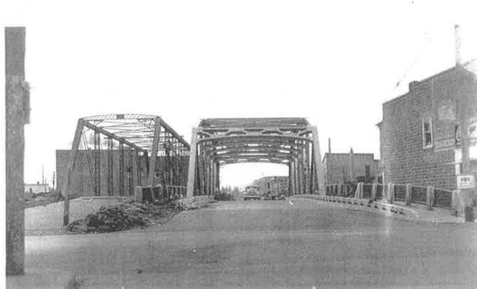
Figure 4. Sheridan Bridge, with 1911 span moved off alignment, Looking South, 1939 (Yamhill County Historical Society)
