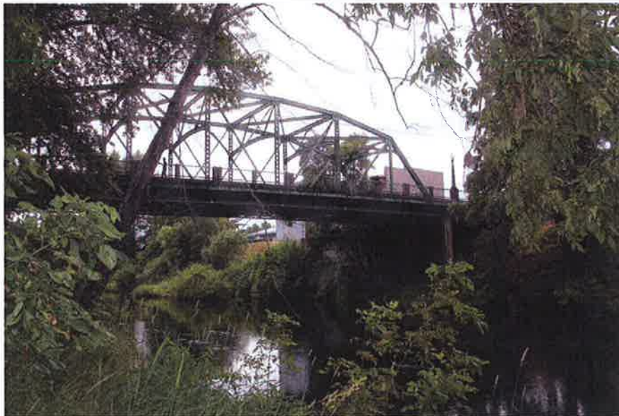
Sheridan Bridge, Looking NW, from Chester J. Moore Park (July 2011)
