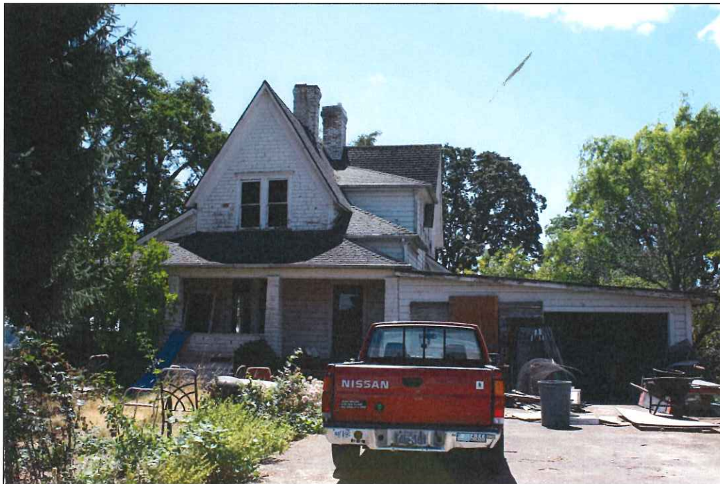
Front (south) facade, looking north
