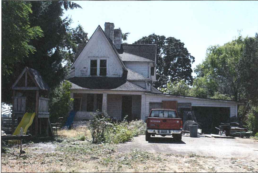
Front (south) facade, looking north
